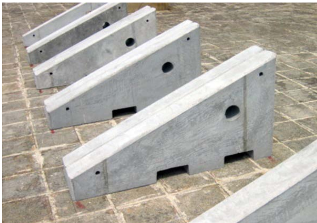
Fig. 11 - Concrete block for PV modules support
