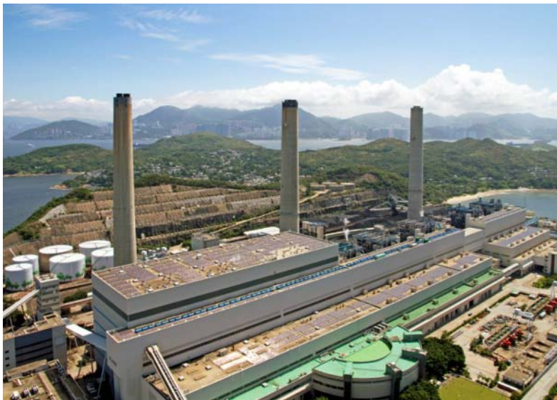
Fig. 4 – Aerial View of Units 1-8 Main Station Buildings and PV System
