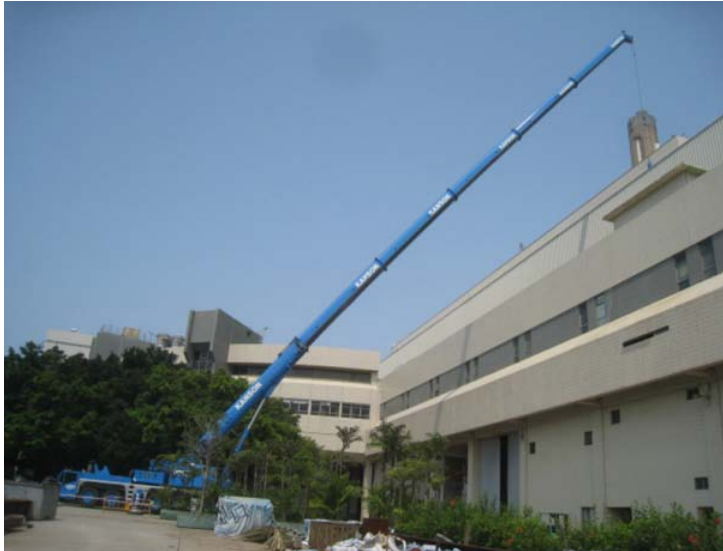
Fig. 13 - Lifting of materials by 250 tonne crane
